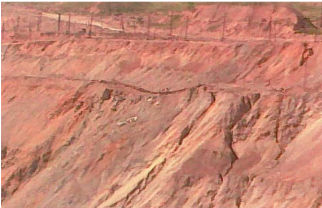
Fig.2. Deformation (landslides-screes) of the southwestern side of the Kalmakyr quarry.
