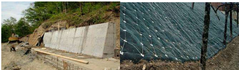
Figure 4. Artificial structure against landslides in mountainous areas.
